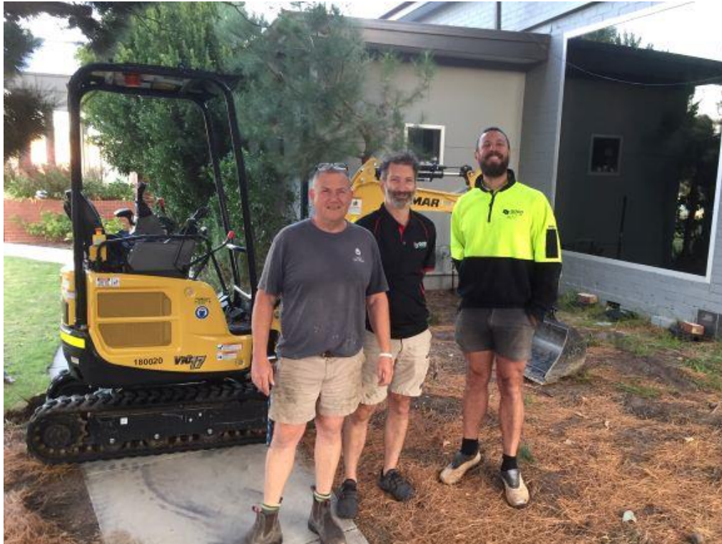
Construction began on 17 March 2021- [L-R Digby Roberts, Clint Woolcock, Ralph Massie]
